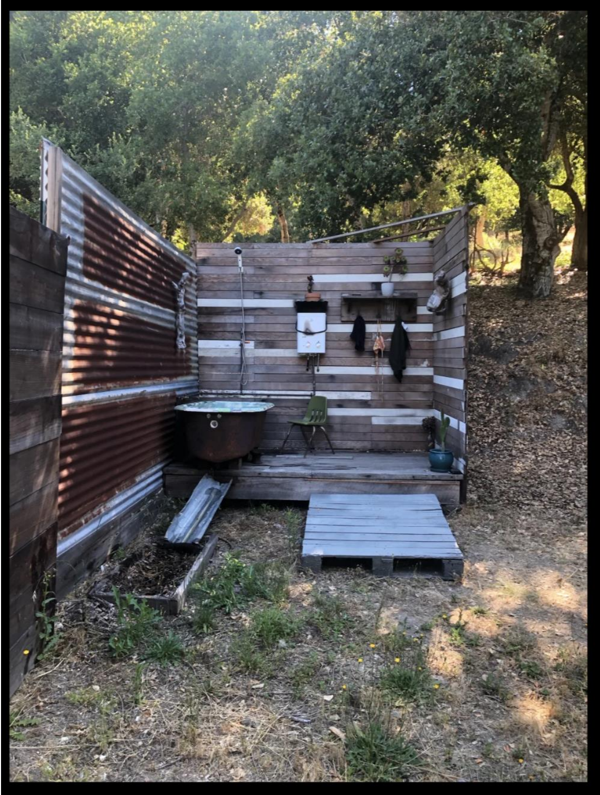
Figure 8d. Outdoor bath with propane heater and water draining on ground. Code requires grey-water systems to drain underground, except for washing machines.
