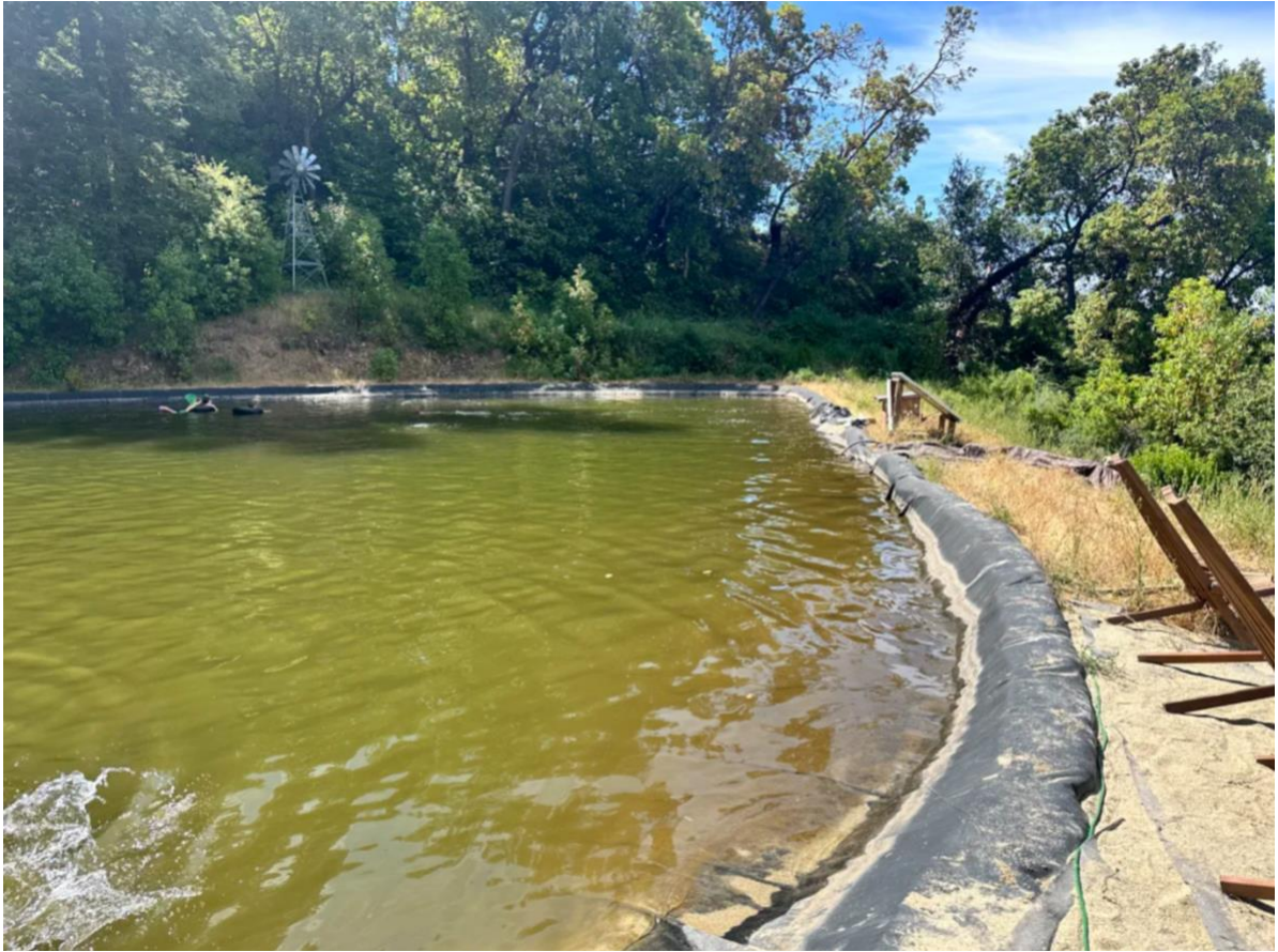
Figure 8c. Artificial pond. Excavating, compacting, and filling soil to create a pond requires a grading permit and a design by a CA licensed professional engineer, registered civil engineer, or registered engineering geologist.
